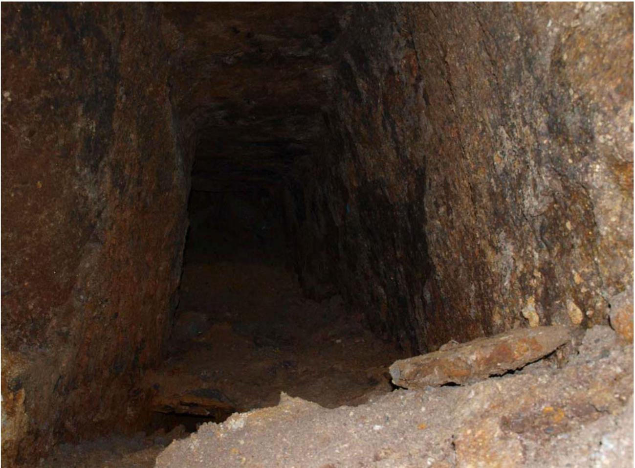
*Fig 12 Roman trapezoidal gallery in Păru Carpeni, with working marks on the walls and roof showing how the gallery was advanced a few centimetres at a time.*
