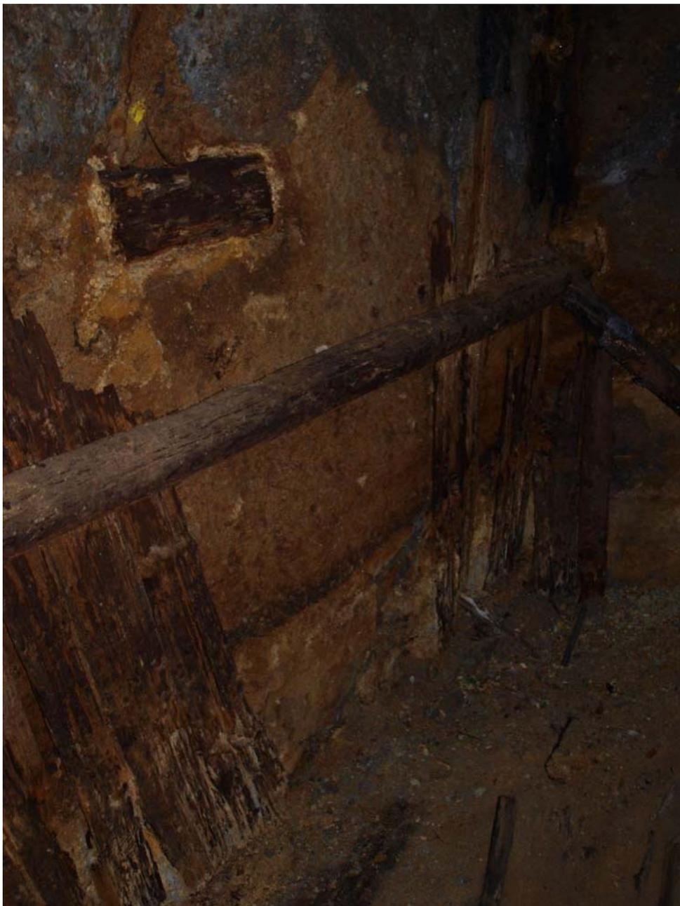
*Fig 17 Păru Carpeni – chamber for a wooden drainage wheel in the Roman mine network. The wooden bearing block for the wheel axle is visible towards the top of the picture, and Roman wooden shoring towards the bottom.*
