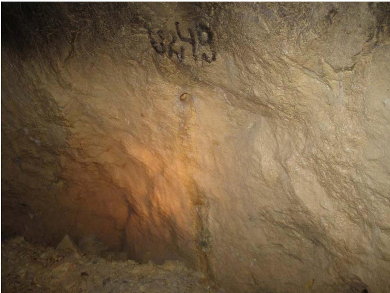
*Fig 18 Shothole for explosive charge in the wall of an early modern mine gallery in the Cărnic massif.*
